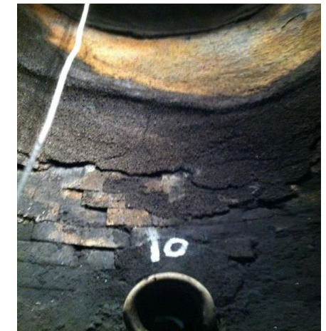
Melt zone after 400,000 tons
